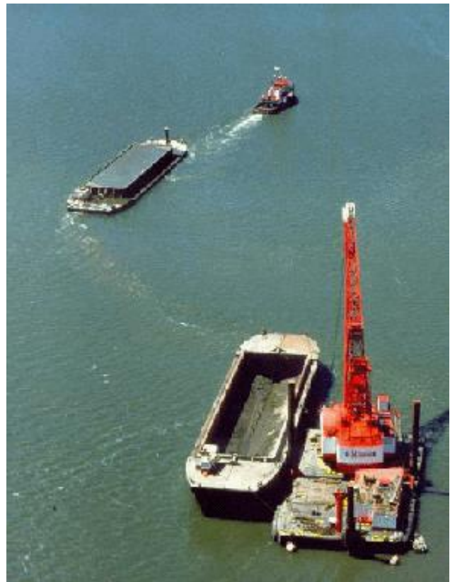
Removal and transport of contaminated bottom sediment
