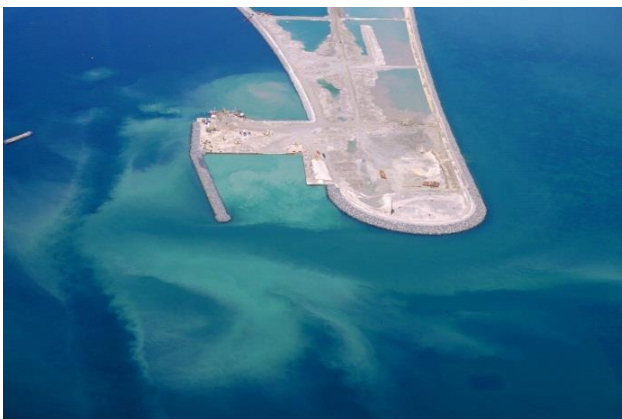
Change in the bathymetry by dredging of the seabed and reclamation of the artificial island 'Peberholm' in Øresund, Denmark
